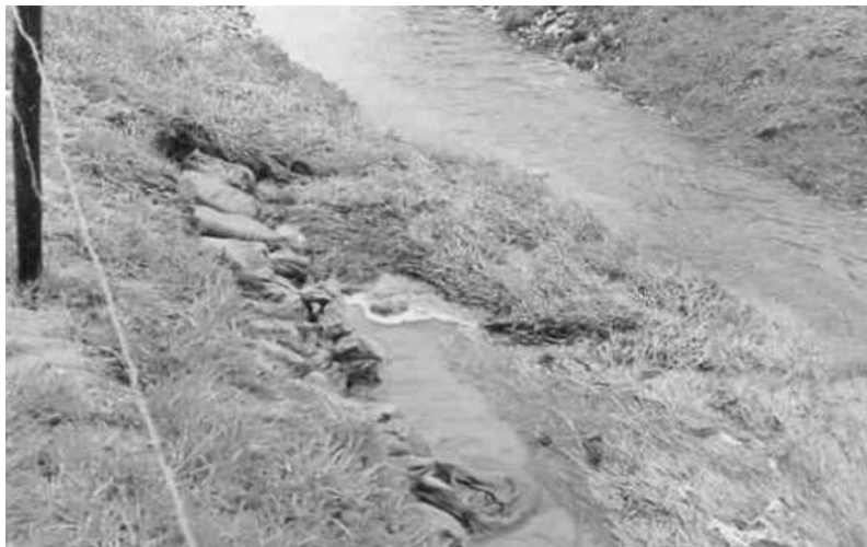
Piping through Embankment
