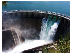
Kerr dam on the Flathead river, U.S.A.
